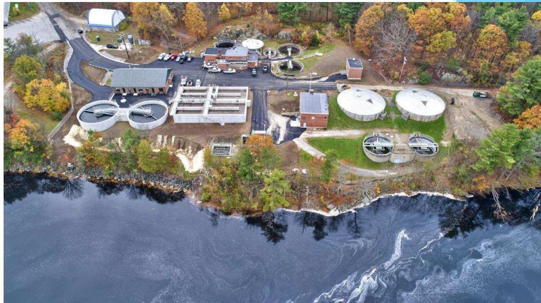
wastewater assets nh - Bing images
