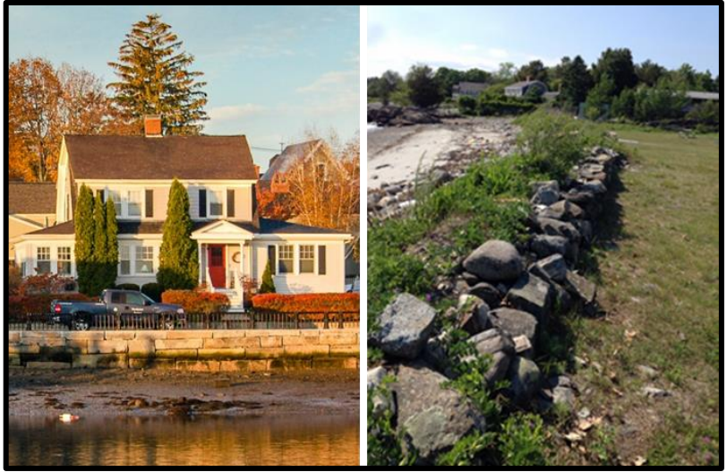
Figure 4: The picture on the left is an example of a concrete sea wall, while the example on the right is an example of a stone wall.
