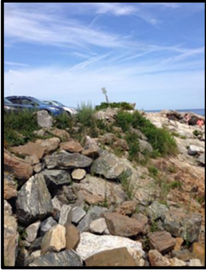
Figure 3: Example of a rip rap structure.
