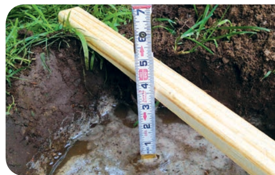
Figure 2 – An infiltration test is performed to determine how well the soil will absorb and infiltrate runoff.
